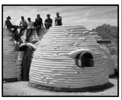
Laborers sit on top of a coil of superadobe tubes formed into a dome. Barbed wire holds each layer in place.
