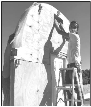
On Memorial Day weekend, Robert Majors (above) helped the Water and Solidarity Collective build a "Conestoga Hut" for a nearby homeless encampment. The hut has a solid, arched front and back pieces with a solid floor; flexible insulation and wire mesh are wrapped around the arches forming the walls and roof. The hut was built in the Catholic Worker backyard and transported on our trailer to the homeless encampment.
