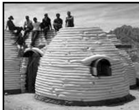
Laborers sit on top of a coil of superadobe tubes formed into a dome. Barbed wire holds each layer in place.
